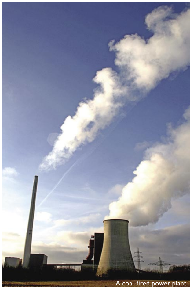
A coal-fired power plant
